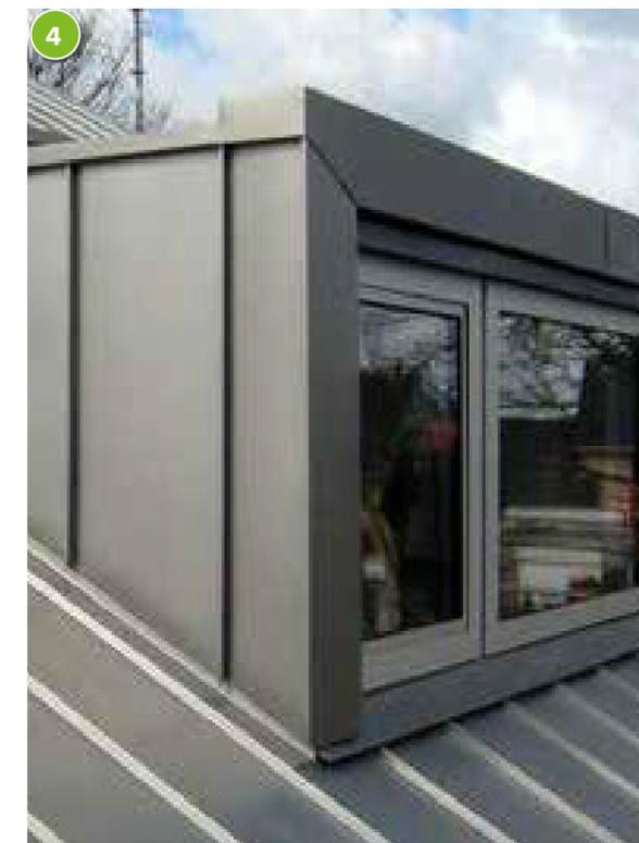
Powder coated (Grey zinc colour) standing seam pressed metal panel finish to box dormer roof detailing.
